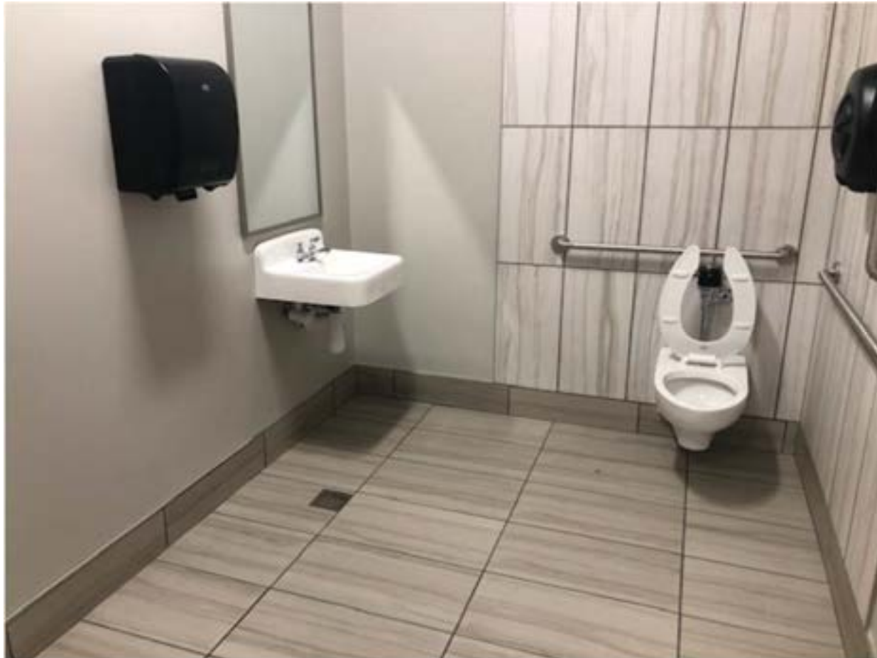
First Floor Progress Photo
