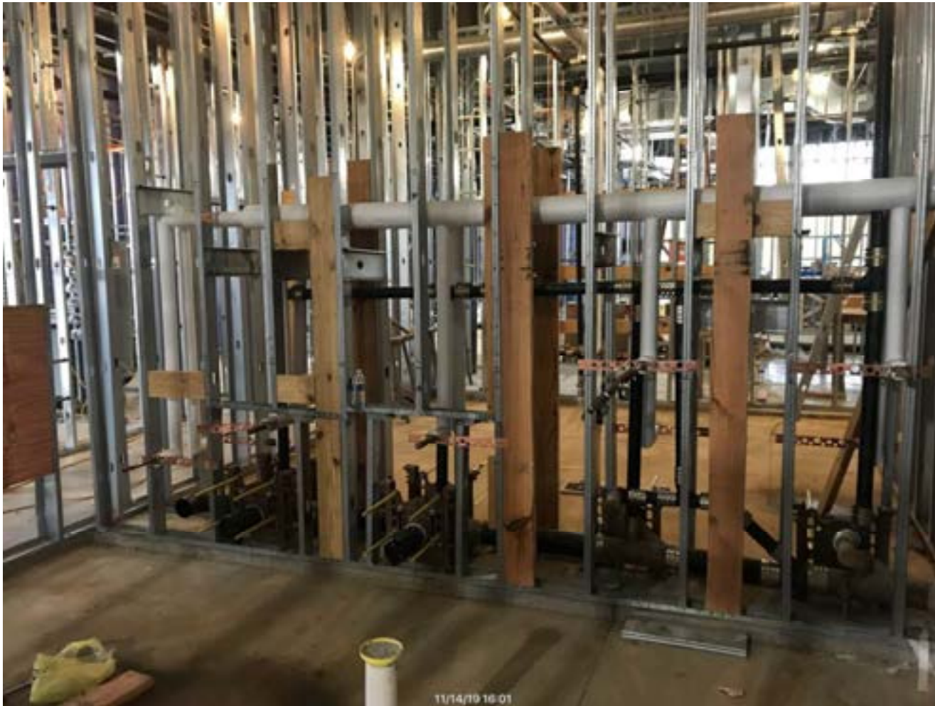
Complete First Floor In-Wall Plumbing Rough-In
