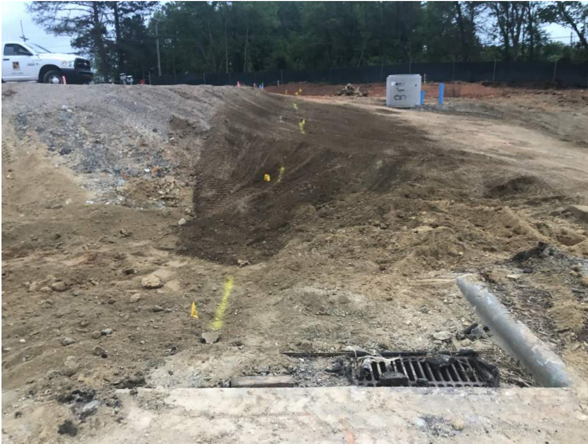
Relocated Gas Line
