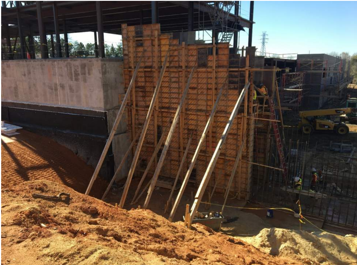
Concrete Wall Forms for Amphitheater Stairs
