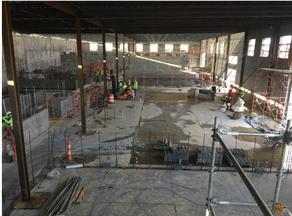
Plaza Level Looking Down from the Mezzanine
