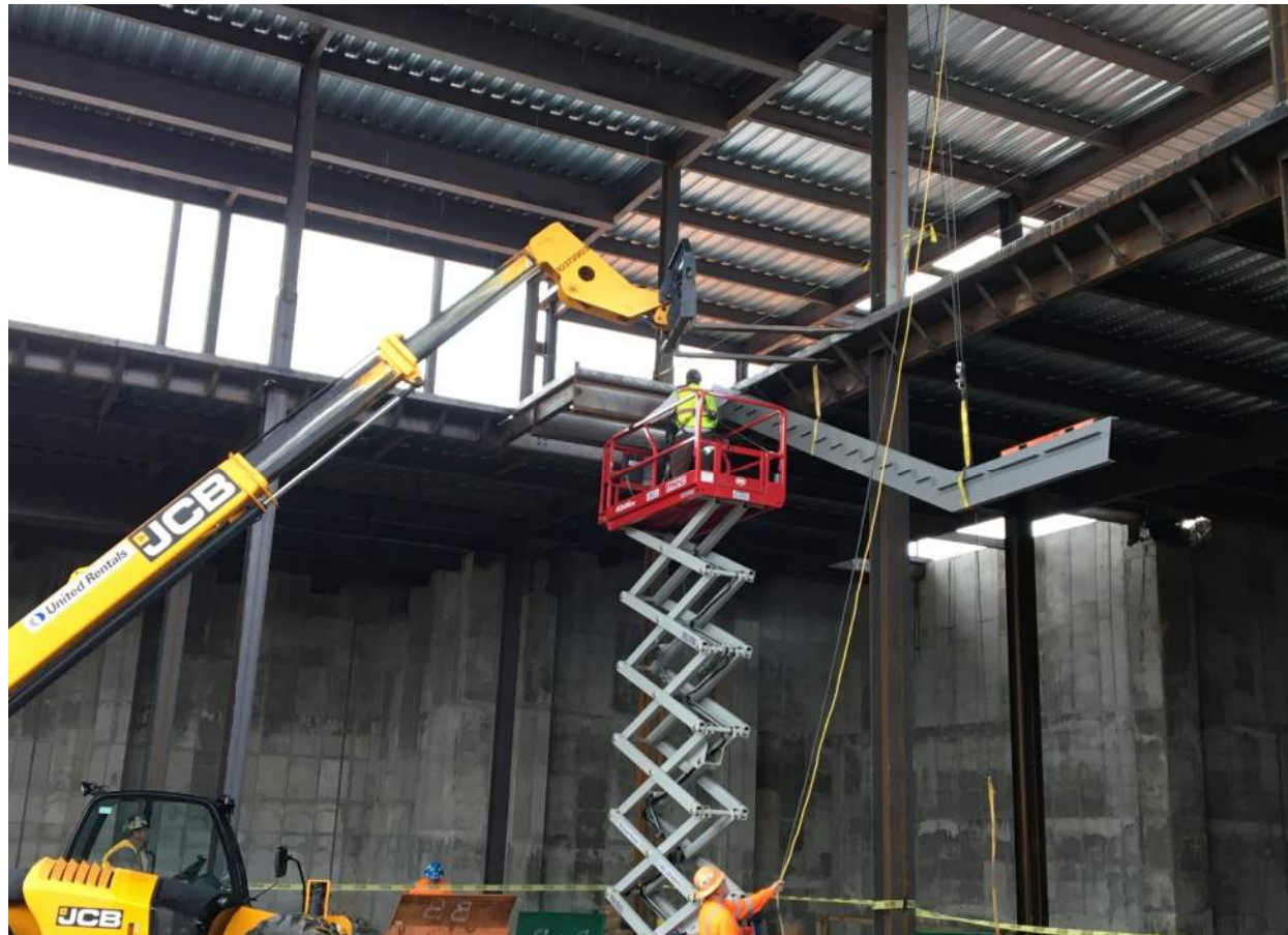
Installation of Stringers at Monumental Stairs
