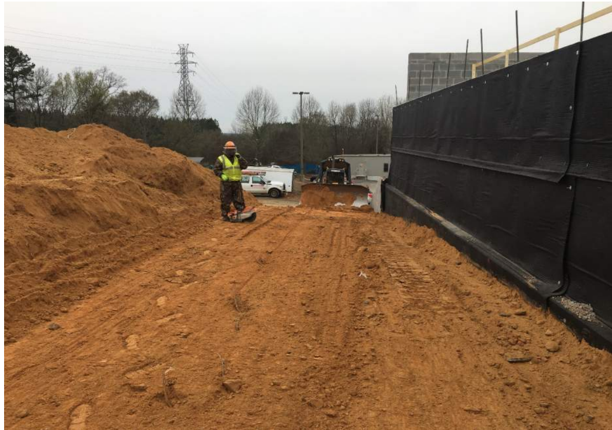
Continuing Backfill Along "8" Line and Soil Nail Wall.
